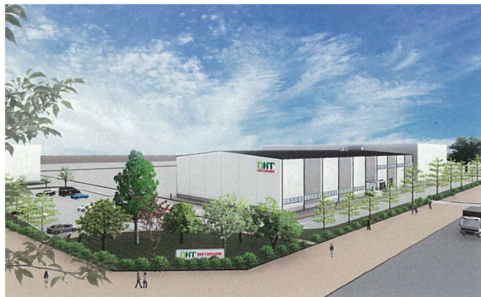
Image of Completion (Construction started in September 2021, scheduled to start operations in FY2023)
