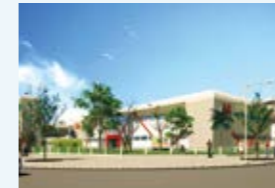
Image of completed factory in Vietnam (Start of construction in November 2021, start of operation scheduled in July 2023)
